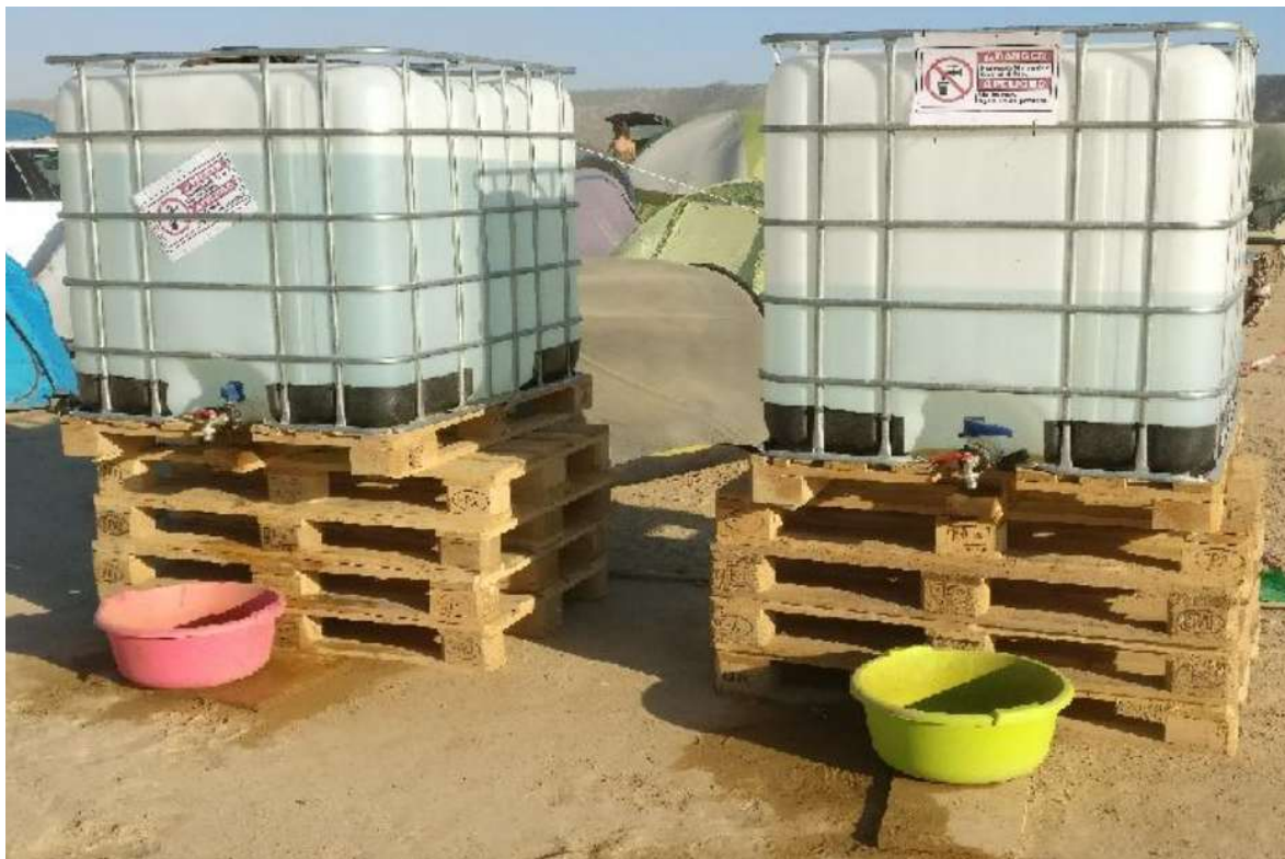
Figure 4: Water cube stand using pallets
